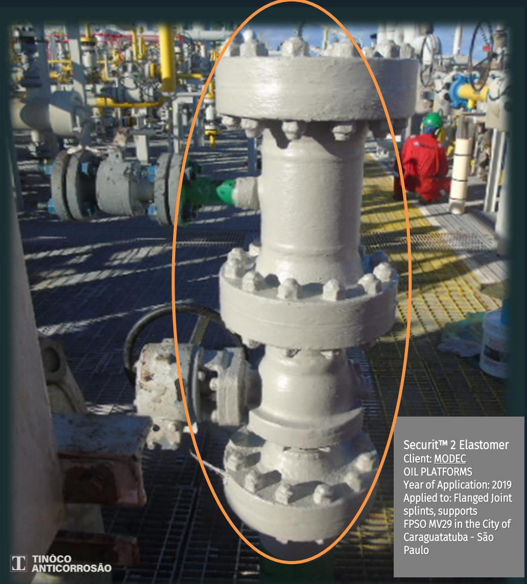
The Securit™ 2 Elastomer Coating System was developed and formulated to offer barrier corrosion protection in areas, equipment, metallic structures and interfaces between steel and concrete, in very high humidity areas. The Securit™ 2 Elastomer has been formulated with state-of-the-art polymers and combined with additives that ensure corrosion protection and waterproofing. This is specially indicated for the protection of areas and equipment under special conditions, such as:
