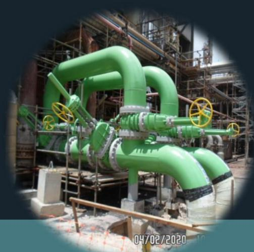
"It's been five years without any type of corrosion, which is a breakthrough in corrosion protection coatings. The application of the Securit™ 2 Elastomer system took place in June 2015 in a CX - Extreme Corrosivity class of aggressiveness - at the BRASKEM plant at the Camaçari Petrochemical Complex site in the state of Bahia(...)"
