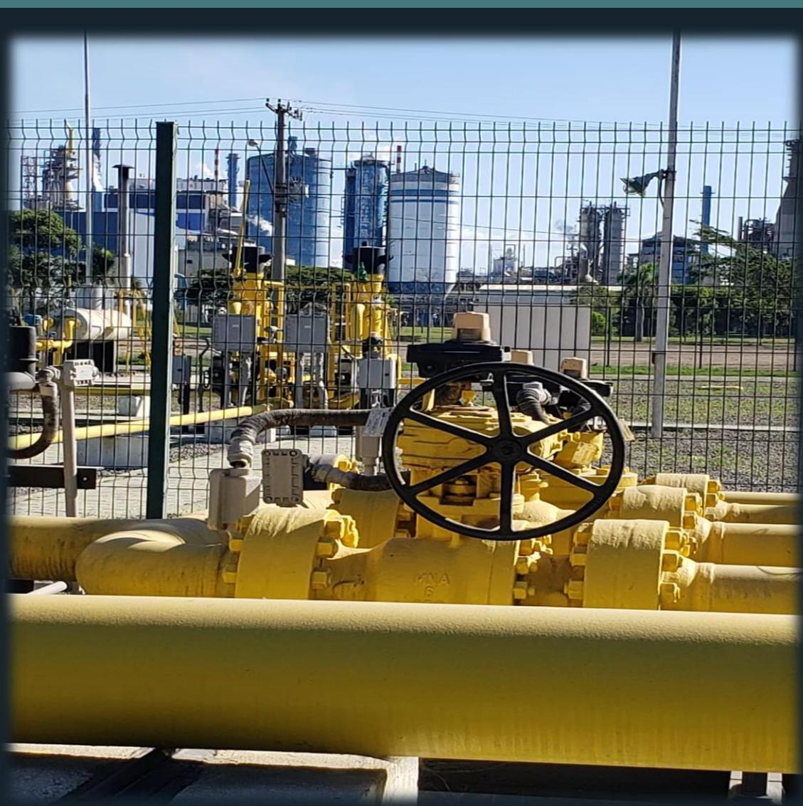
Application of the Securit™ 2 Elastomer in CRITICAL AREAS OF THE SITE which were exposed to both: atmospheric and galvanic corrosion:
