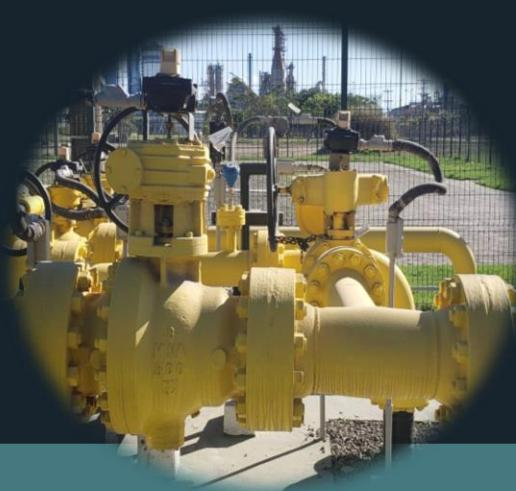
"Under my supervision, the company RIP / KAEFER performed the maintenance and painting services of the ARCEL ERP unit. We found all flange joints coated with Securit™ 2 Elastomer in good sealing condition and without onset of corrosion. There was no need for maintenance/ repair. We only applied a top layer of yellow liquid polyurethane-based paint to reinstate the surface gloss and aesthetics of the elastomeric coating system after 7 years exposure following from its original application"
