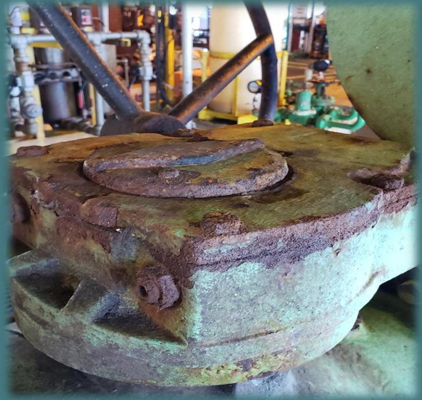
The durability of the infrastructure assets of the industries is reduced by the action of corrosion that is accelerated by: the presence of pollutants in the atmosphere, high relative humidity, marine atmosphere (Sodium chloride salts) and high temperature.
